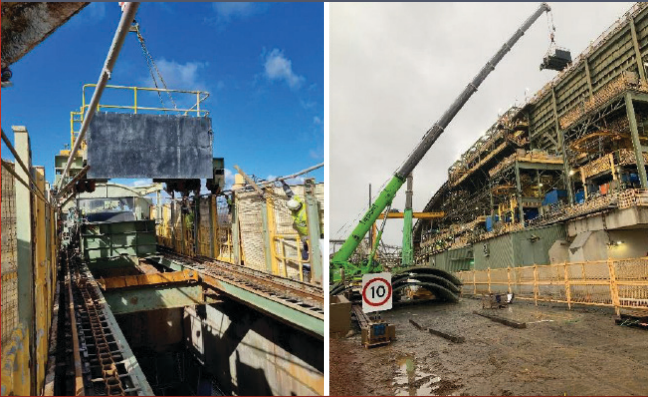
Replace Shuttle and Sweeps
