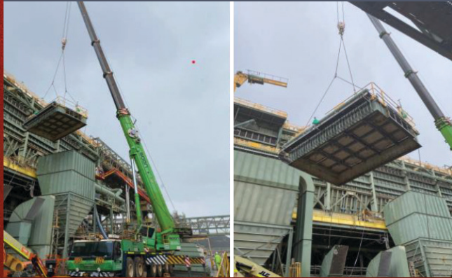
Replace HPGR Baghouse
