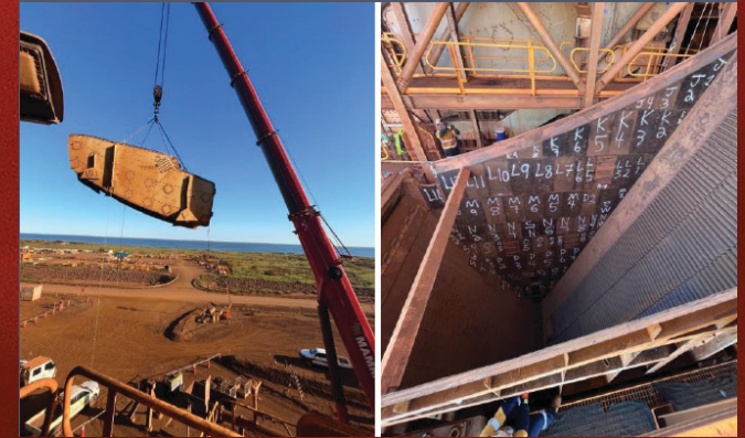
CLB Screen House Upgrade
